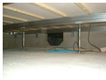
Fig. 2. Typical under floor of the Japanese house.
