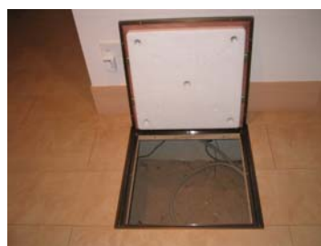
Fig. 4. Inspection hole installed on the floor.
