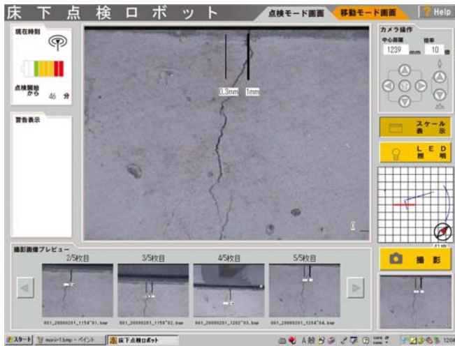
Fig. 12. Human interface of “inspection mode” for crack width measurement.
