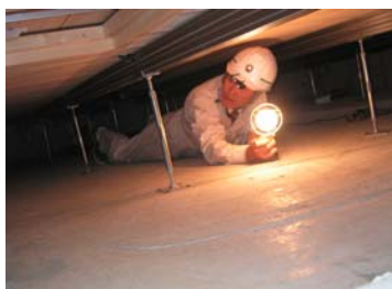
Fig. 1. Inspection of under floor of house by human.
