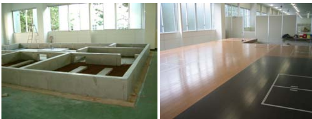
Fig. 13. Test field. Before covered (left) and after covered by floor(right).
