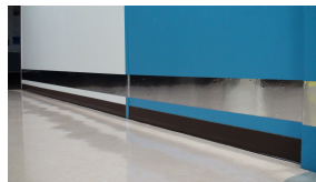
Fig. 8 Setting position of mirror tape
